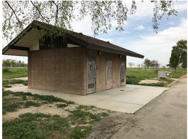
Restroom and Fish Cleaning Station
