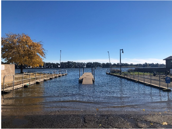
Boat Ramp and Pile-Guided Boarding Float
