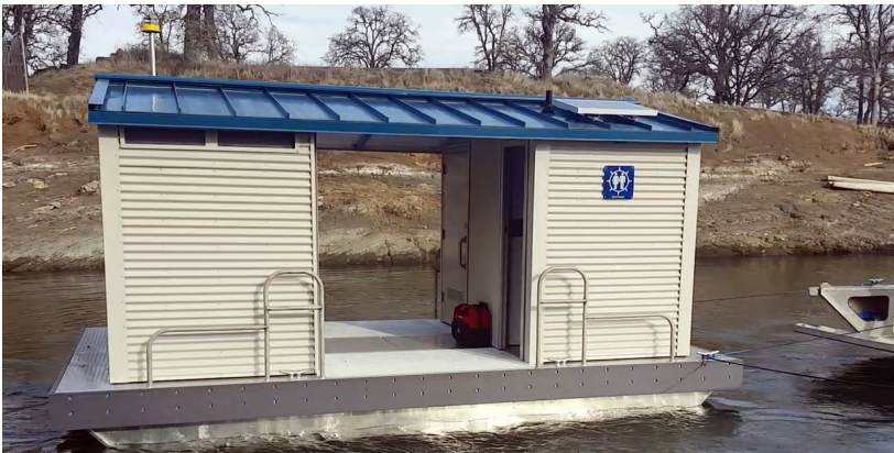
Floating Restrooms in Lake Berryessa
